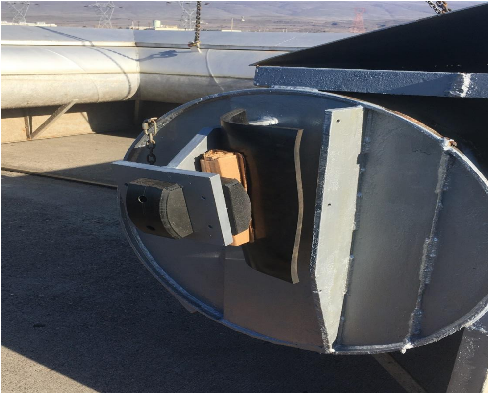
New rubber seal for oil barrier on north exit debris guard
